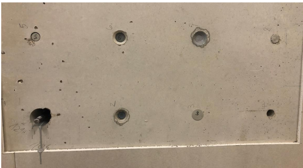
Fig. 10: Detail of form-tie points 1 to 8 of side 1
