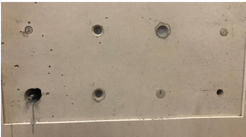
Fig. 10: Detail of form-tie points 1 to 8 of side 1
