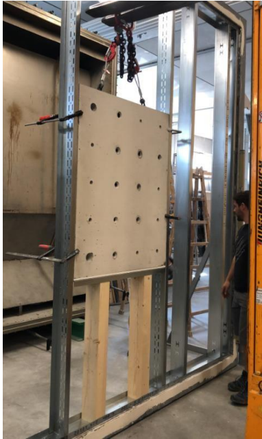
Fig. 8: Installation of the concrete block (side 1) in supporting construction
