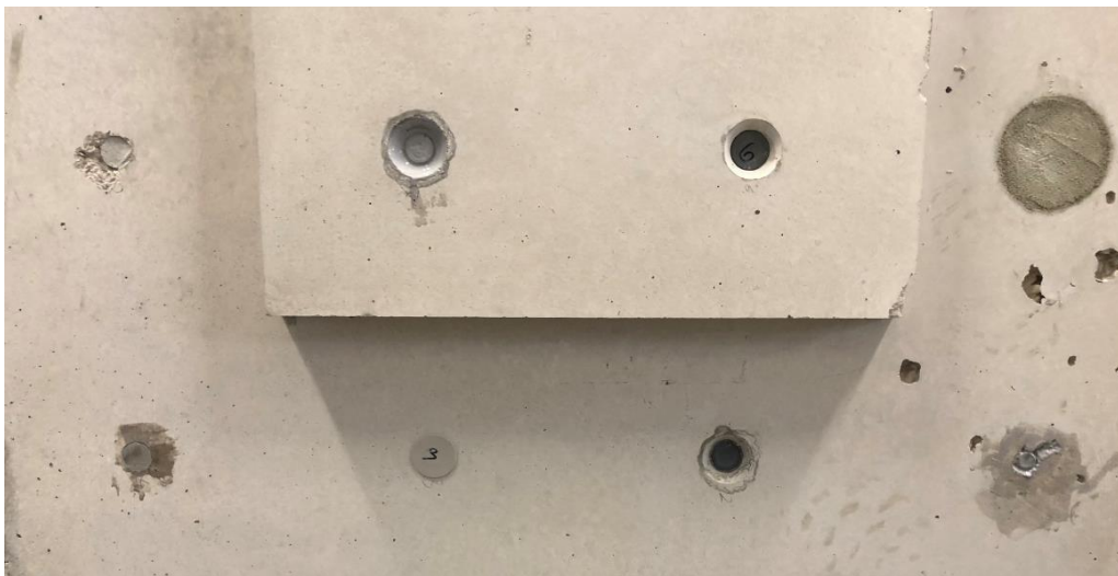
Fig. 12: Detail of form-tie points 1 to 8 of side 2
