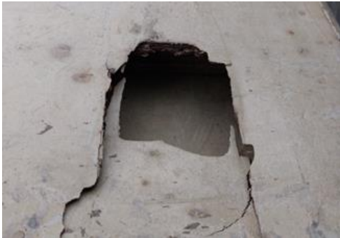
Holes + drills diameter > 2 cm
