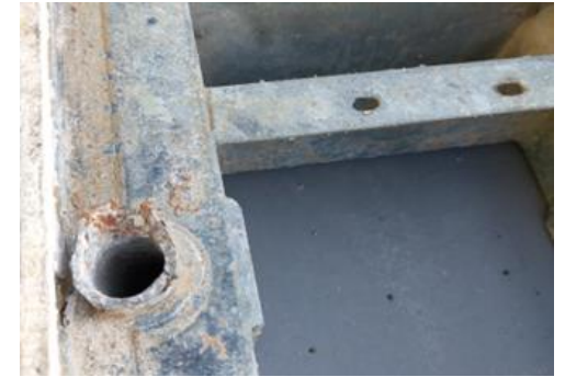
Missing or damaged anchor protection
