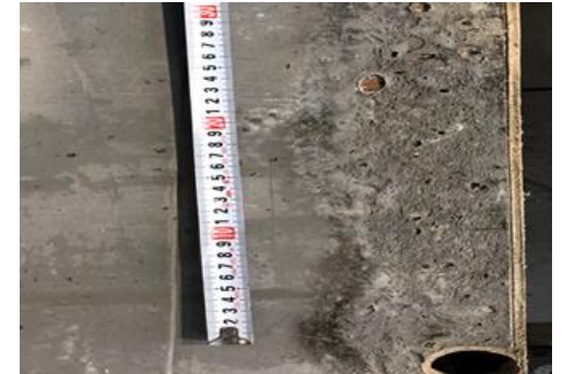
Burned plywood = 10 cm
