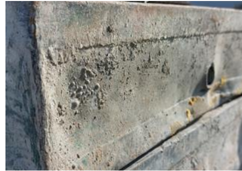
Frame profile dented
