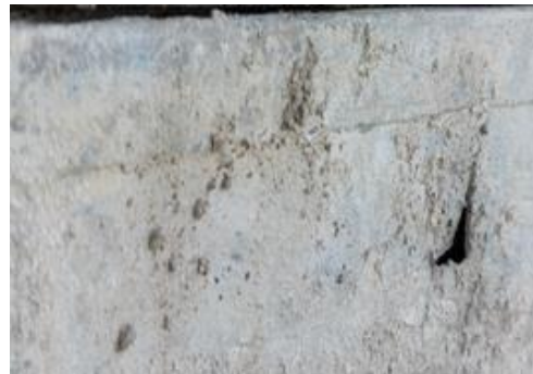
Hole in profile – weld needed
